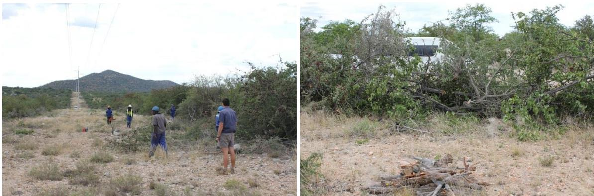
**Figure 11: Maintenance team busy clearing a transmission line servitude**
